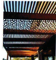
10 OVERHEAD STRUCTURE AT ENTRY GATE
