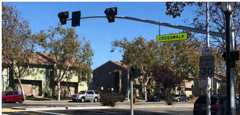
A newly install pedestrian hybrid beacon installed as part of the Yellow Brick Road project at Barrett Avenue/8th Street.
