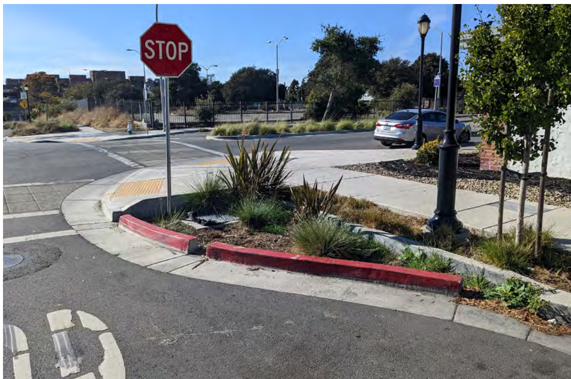
A curb extension with green, stormwater infrastructure near the Richmond BART.
