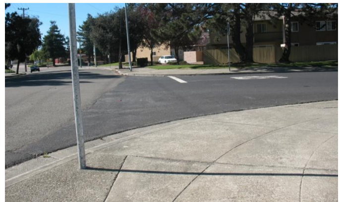
Missing curb ramps and wide corner turning radii, Bayview and Ellis
