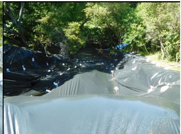
Photograph 11. Fence and Tree fall into slide on 3/30/2023. Photograph 12. Tree partially removed and slope recovered with plastic sheeting as seen on 4/10/2023.
