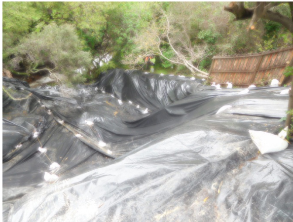
Photographs 9 and 10. Landslide covered in plastic sheeting on 3/14/2023.
