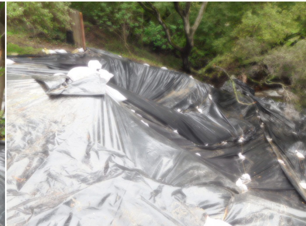
Photographs 9 and 10. Landslide covered in plastic sheeting on 3/14/2023.
