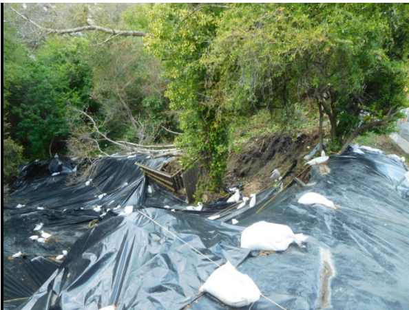
Photograph 11. Fence and Tree fall into slide on 3/30/2023. Photograph 12. Tree partially removed and slope recovered with plastic sheeting as seen on 4/10/2023.
