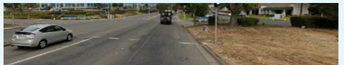
Missing sidewalks near more active land uses
