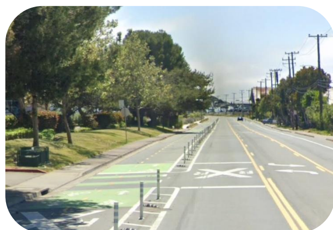
#SB115 Street Paving – SB1 – Cutting Harbour Way S. Bikeway
