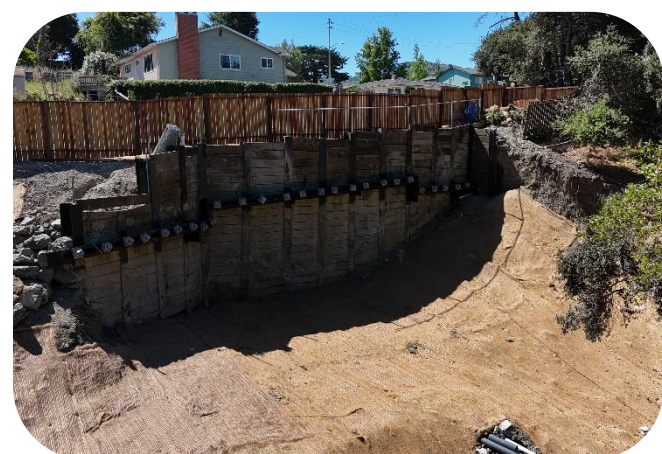
#23037 Santa Rita Road Stabilization
