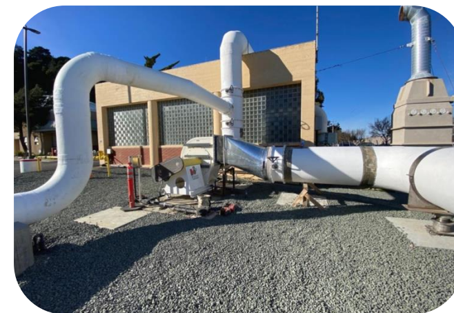
#01X10 Grit and Aeration Replacement
