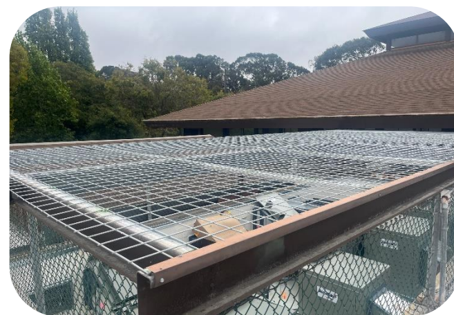
#AR247 Booker T. Anderson Community Center HVAC Renovation (Phase 2)
