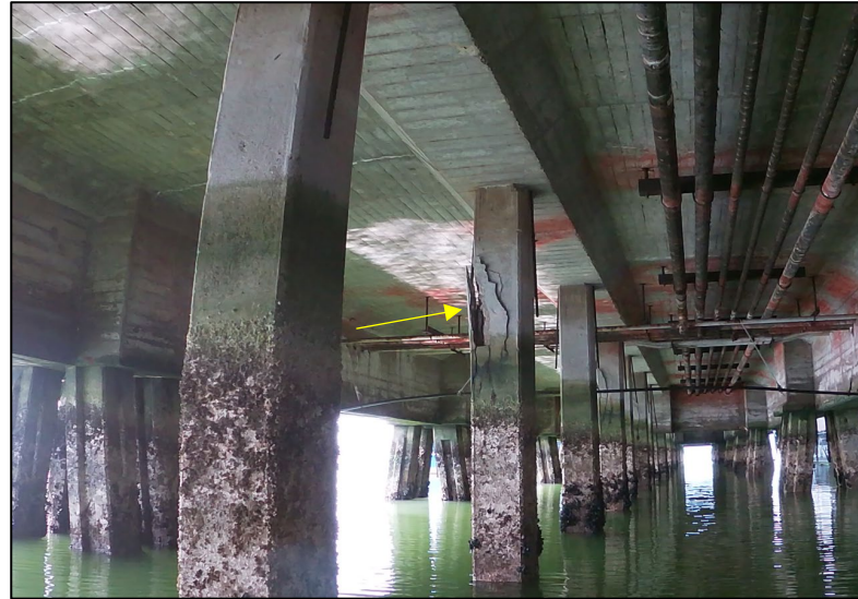
Typical pile damage at internal row
