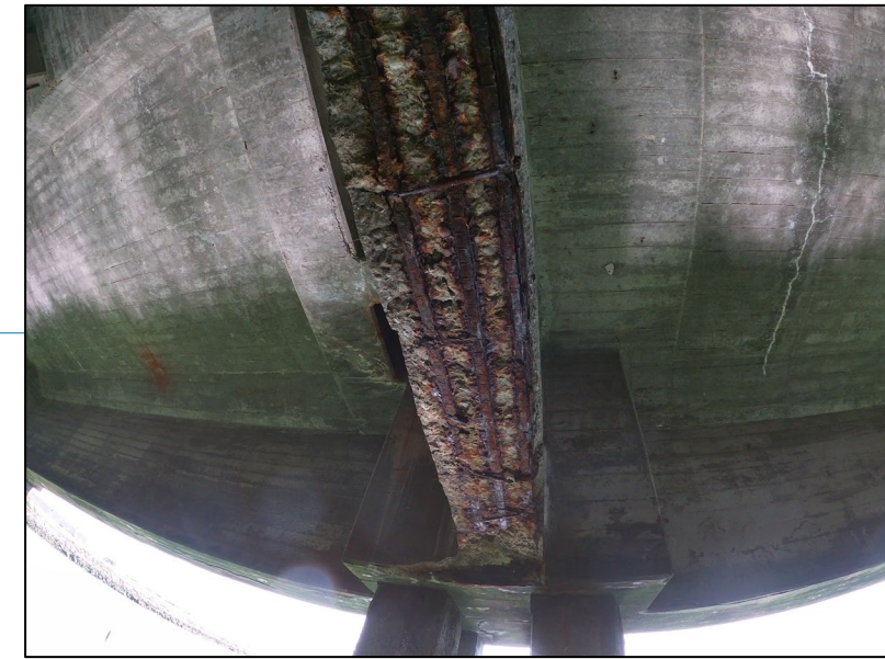
Exposed reinforcing at deep beam
