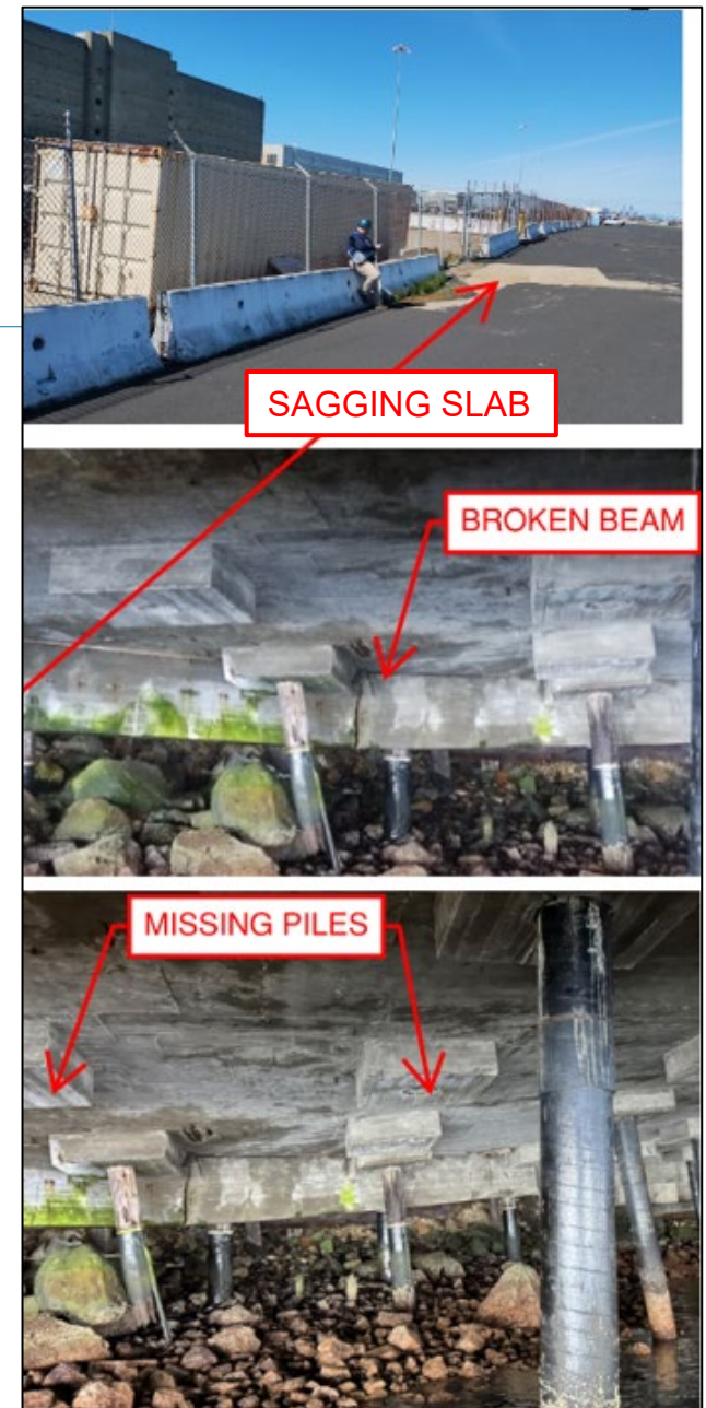
Damage at Berths 5-6
