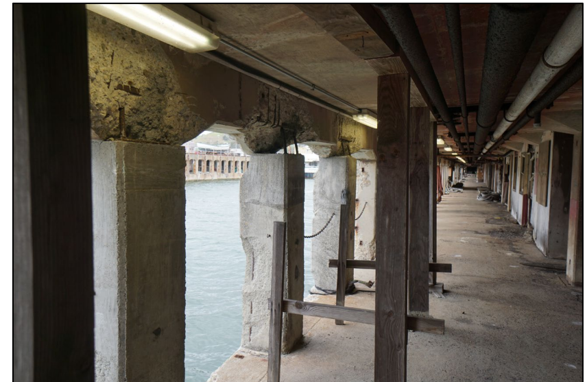
Damage at Berths 7-8 (above) Columns in Serious condition at Graving Basin (below)
