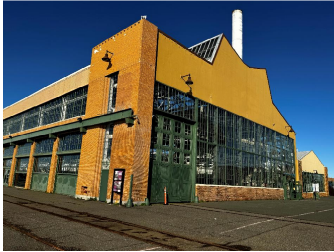
Photo 9: Building exterior from south west visible railroad tracks (1/8/2026)
