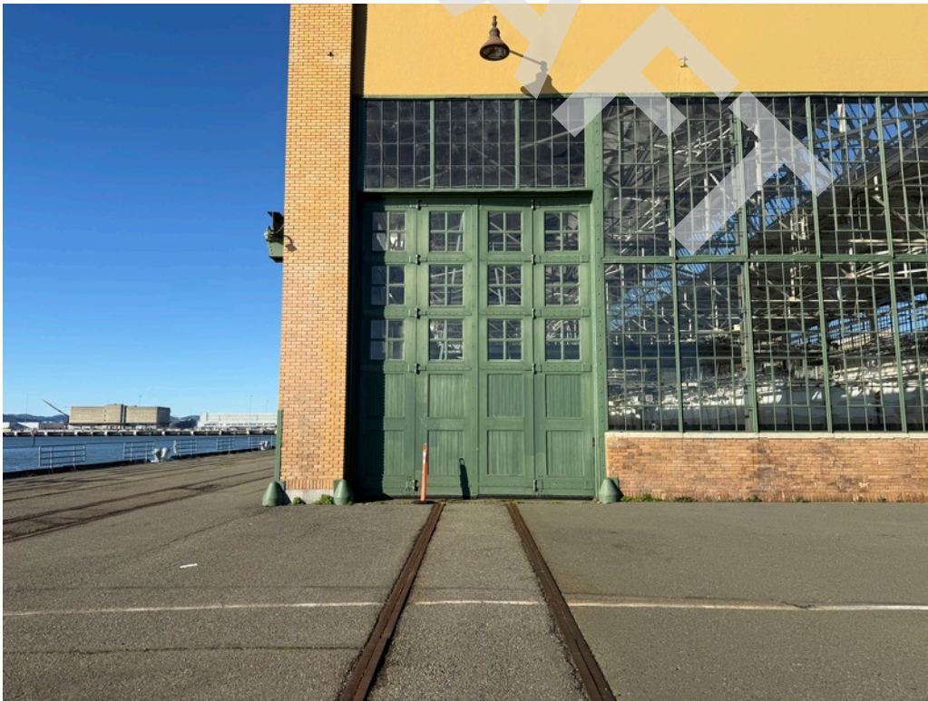
14 - Multi-panel industrial craneway door provided at the east elevation of the building.
