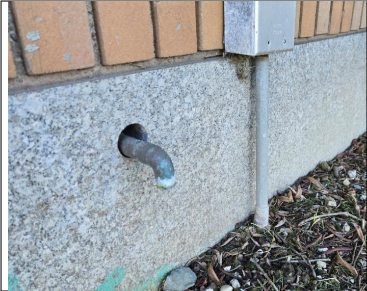
Figure 21. Granite at base of wall
