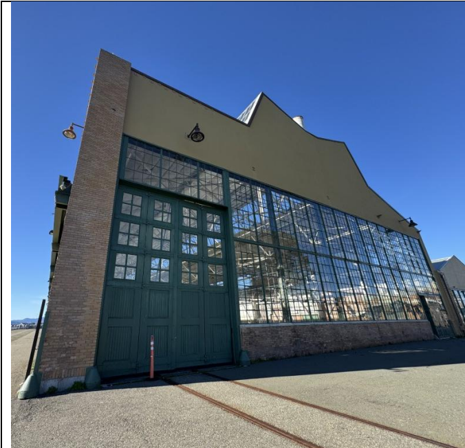
Figure 25. East elevation of Craneway Pavilion, gunite wall above window bay
