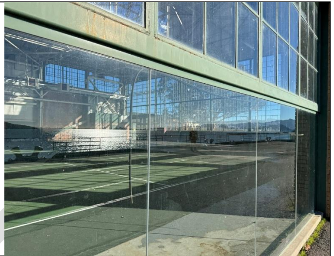
Figure 30. Newer butt-glazed window system on south elevation at ground floor
