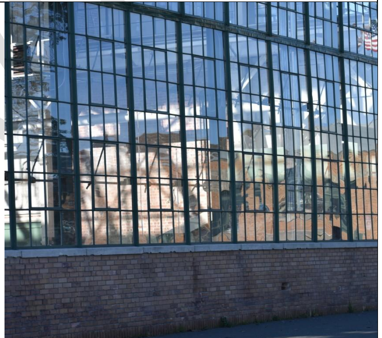
Figure 28. Existing steel-framed single-pane window system
