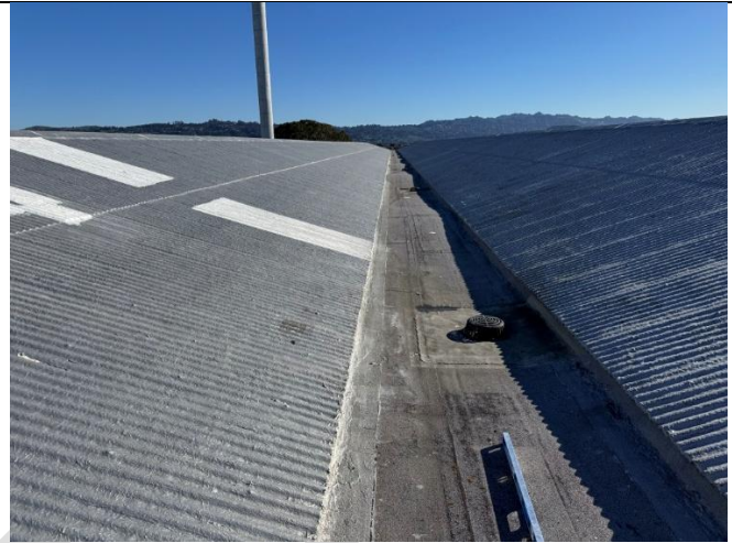
Figure 46. Overview of steep-sloped coated transite roof panels at upper sawtooth roof
