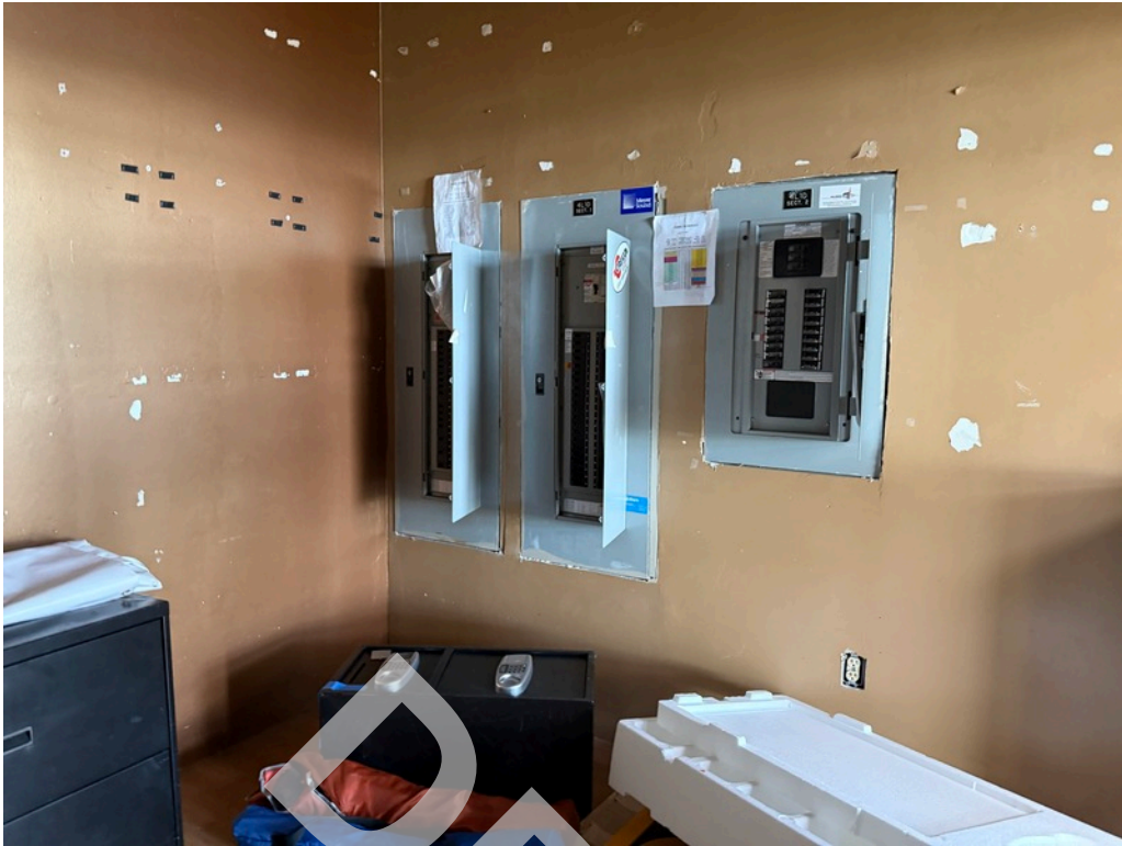
21 - Typical utility room finishes.
