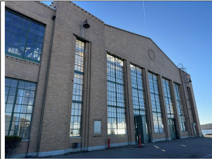
Figure 1. West elevation Craneway Pavilion
