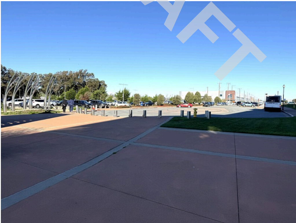
8 - Precast concrete paving is provided at the northwest corner of the site.
