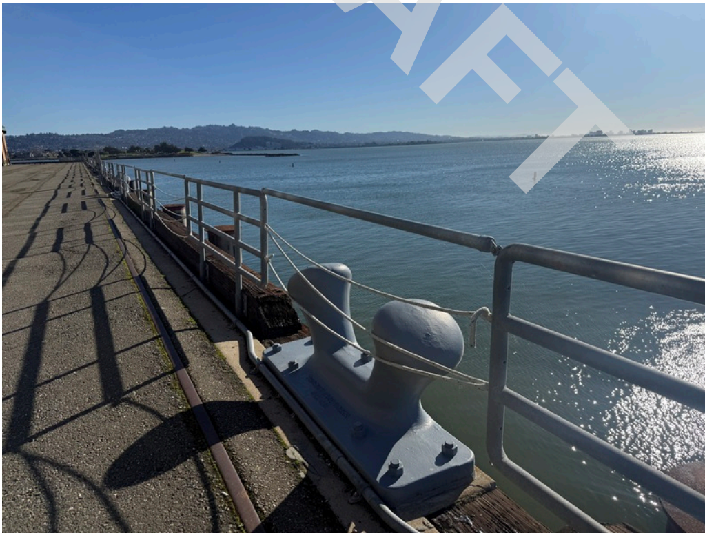
10 - Metal guardrails provided along the south boarder of the site.
