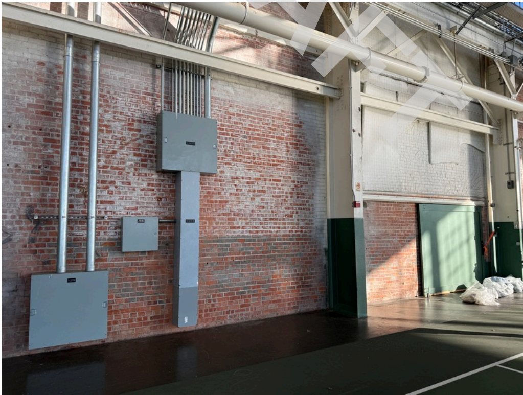
18 - Interior historic brick and mortar walls.
