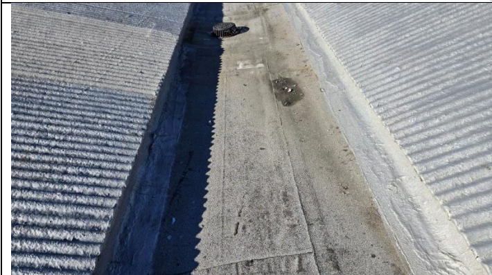
Figure 55. Low-sloped bituminuous membrane at upper sawtooth roof
