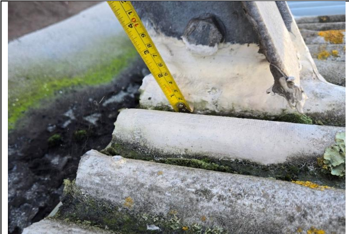
Figure 53. Liquid flashing at parapet brace where penetrating through metal roof
