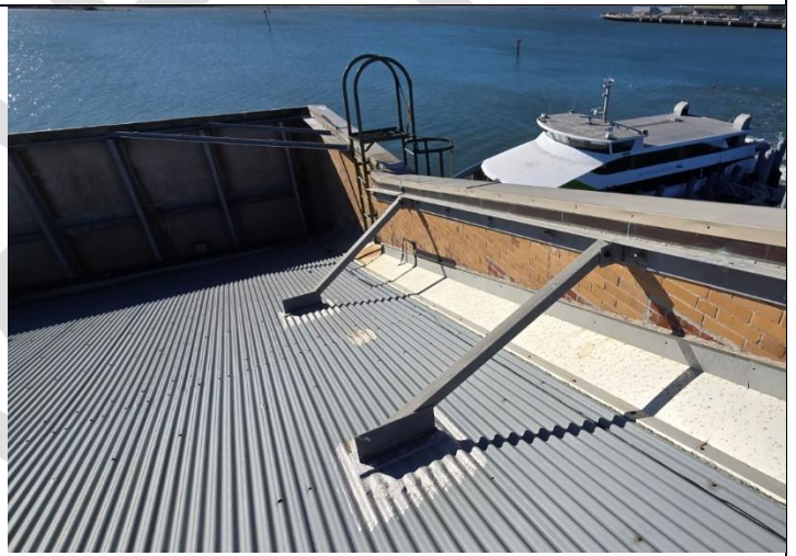
Figure 12. Brick parapet braced back to roof deck
