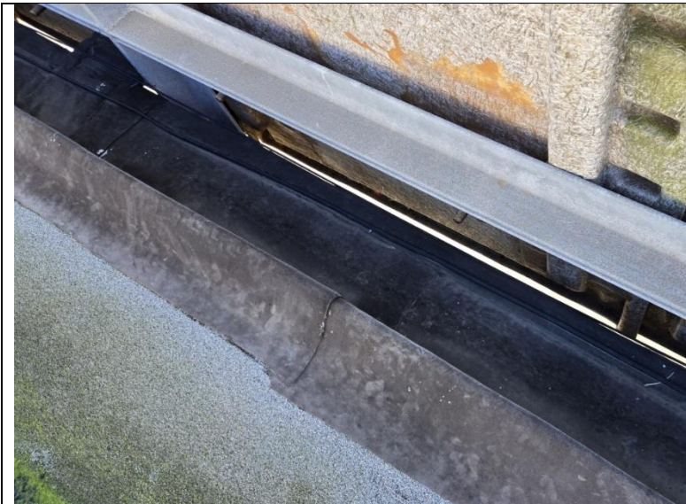
Figure 17. Interface between backside of parapet panelized wall system and SBS/EPDM roof membrane at ledge
