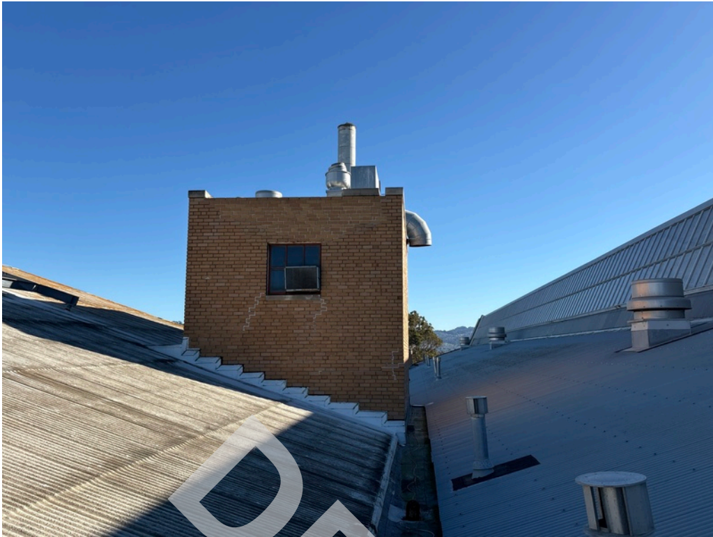
29 - Small Main Building tower projecting above the main roof with HVAC equipment for the service kitchen in the Craneway Pavilion.
