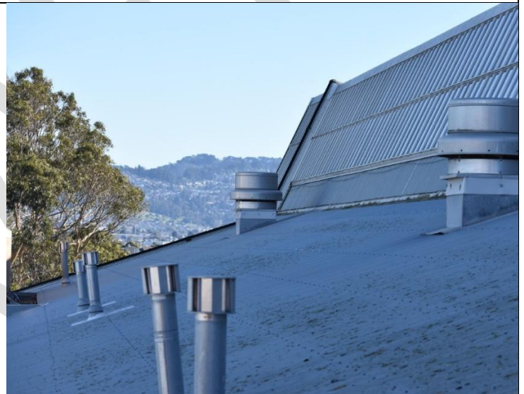
Figure 48. Overview of lower steep-sloped metal roof panels
