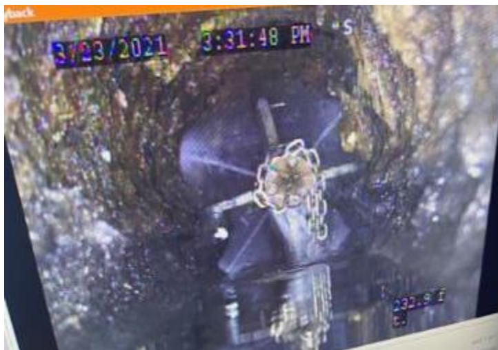
Figure 1. View of Keller Beach sewer pipe prior to cleaning. Hydro nozzle is in use. Chain flail is in view.
