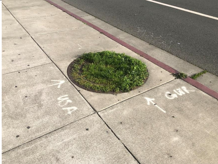
Figure 6 - Example of empty tree well
