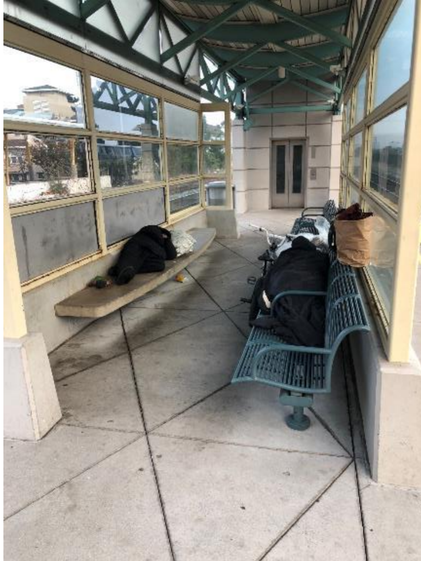
Figure 3 - Waiting area for AMTRAK has become a homeless shelter. Windows are broken and steel frames are rusted and require painting
